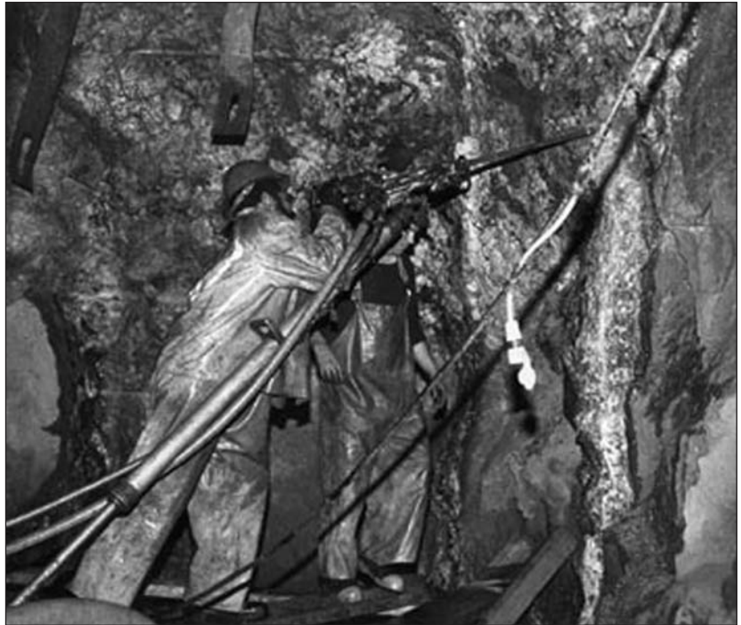
Sandhogs drill into bedrock underground. [Photo source: Department of Environmental Protection]
